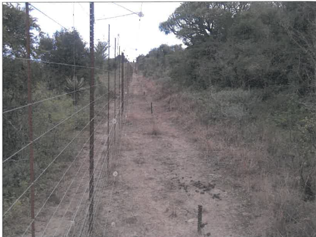
Figure 3: The existing perimeter fence at the GFRNR
