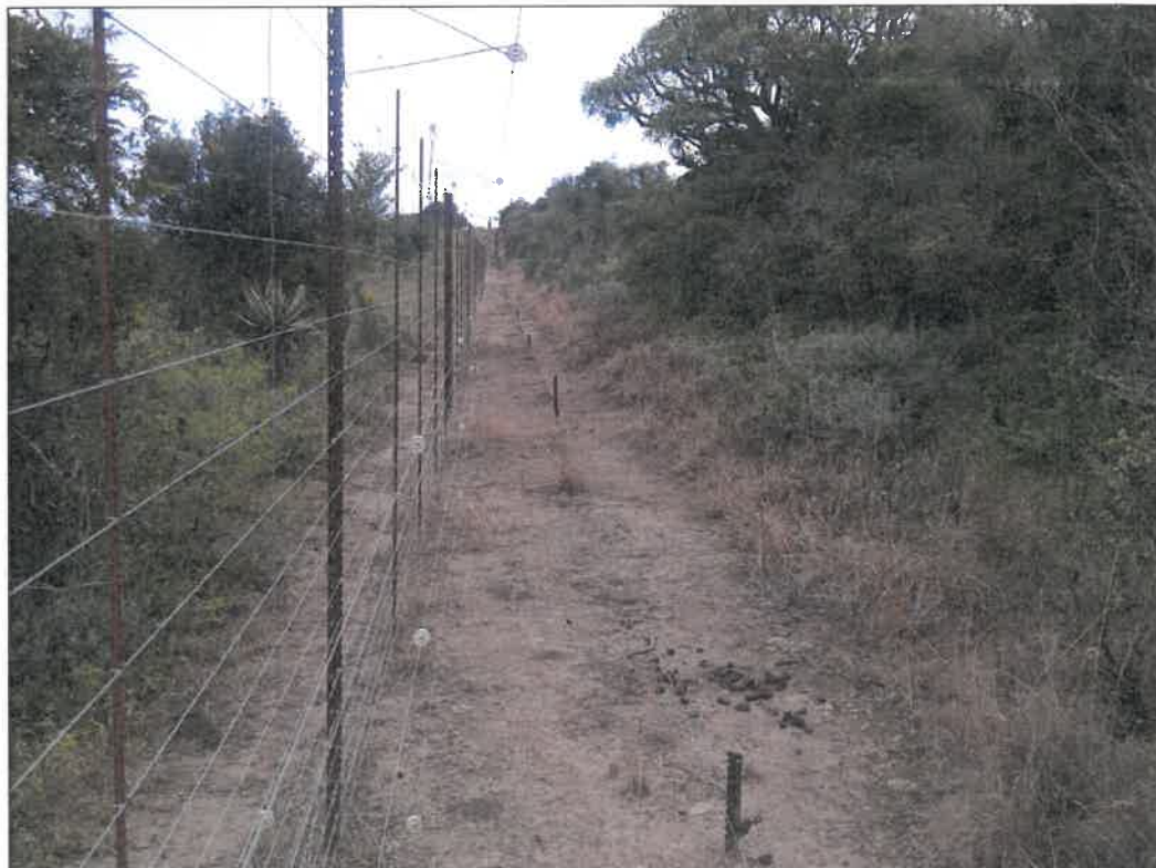
Figure 3: The existing perimeter fence at the GFRNR
