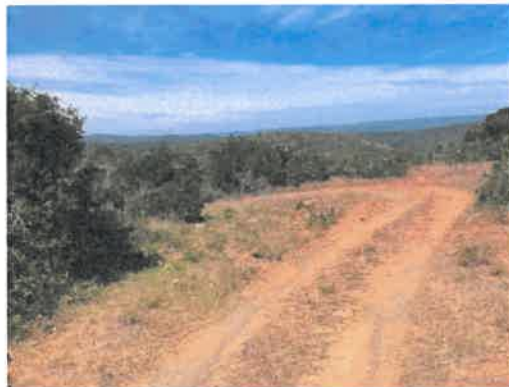
Figure 5: View (1) of an example of the internal gravel roads to be maintained within their existing footprint.
