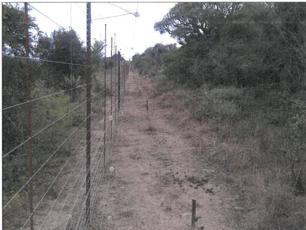
Figure 3: The existing perimeter fence at the GFRNR
