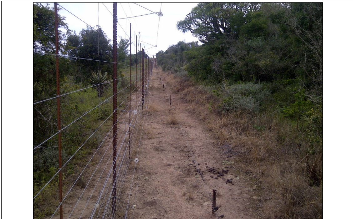
Photo 2-1: The existing perimeter fence at the GFRNR.
