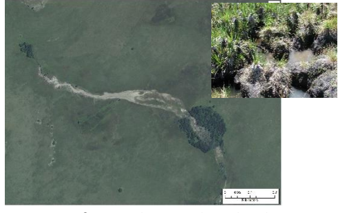
Erosion from a damaged wetland
