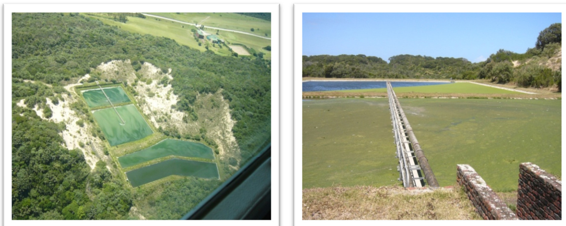
FIGURE NO. 3 Existing Municipal Sewerage Oxidation Ponds
