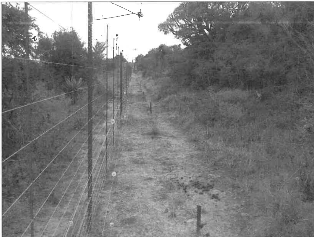
Figure 3: The existing perimeter fence at the GFRNR
