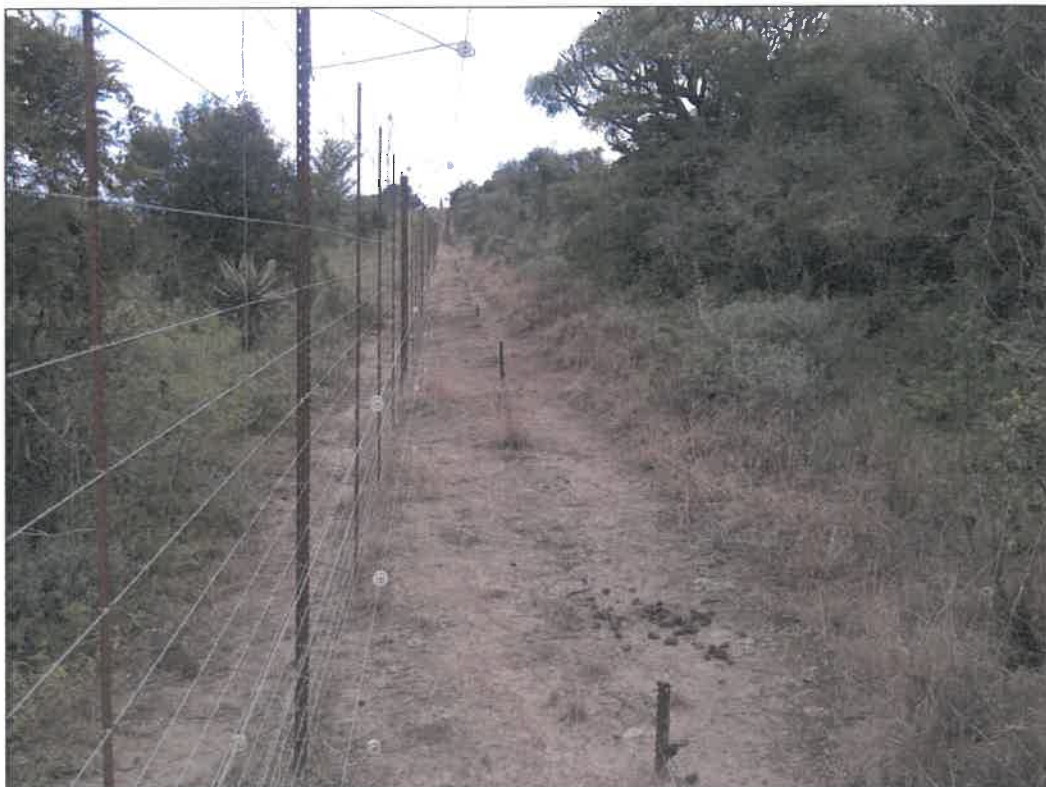
Figure 3: The existing perimeter fence at the GFRNR
